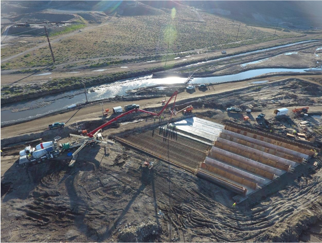
Cast In Place RCB Sta 79
